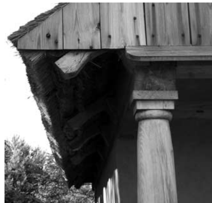
Fig.5 Traditional rural building in the open air museum near Gdansk, Poland. Detail of the connection between the wooden column and the roof.
