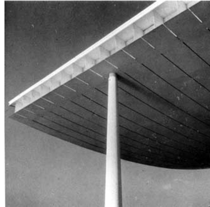
Fig.10 Exposition pavilion at the "Fiera del mare", Genoa, Italy, 1963. Detail of the connection between the concrete column and the roof.
