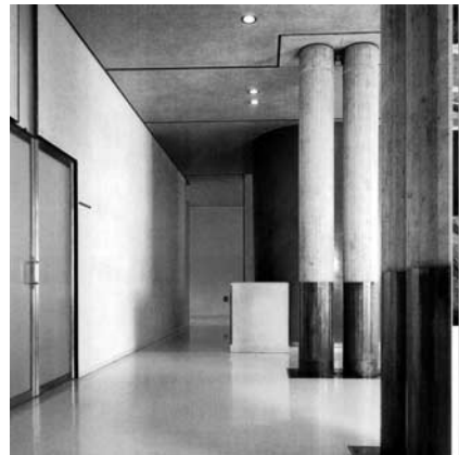
Fig.11 Carlo Scarpa, "Banca Popolare di Verona", Italy, 1973-81. Detail of the connection between the concrete columns and the ceiling.
