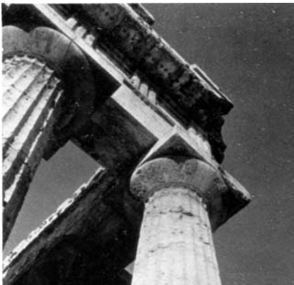
Fig.8 The corner of a Doric temple. Detail of the capital.
