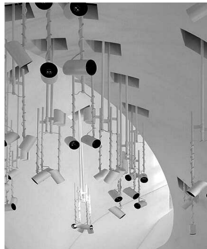
8. Completed committee room ceiling showing lighting interface.
