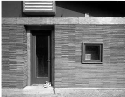
wall made of carpet tiles (Lucy's House -S. Mockbee)
