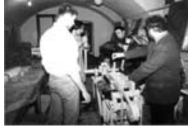
Compressing blocks in hand operated press
