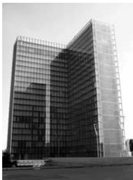
Picture 16: A much appraised and awarded project, which could serve as an example of typical modern architectural ego: Perrault's building, apart from the massive use of tropical wood, also fails to take its own purpose into consideration by endangering books through vast areas of glass.
