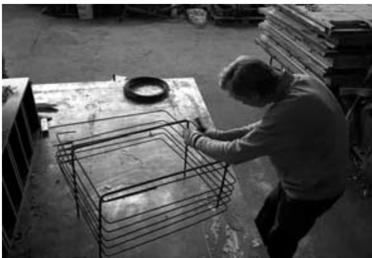
Exercise II Preparing the Steel Reinforcement
