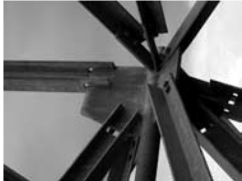
Fig 5B: Acoustic Barrier, ONL [Oosterhuis_Lénard] 2004, File to Factory process of Mass-Customization generates 10.000 different nodes
