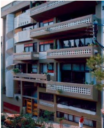
Block of Flats, Benaki Street, Athens, 1972
